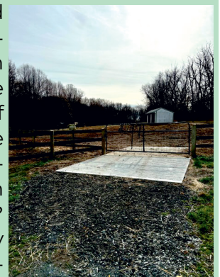
The concrete pad provides a stabilized gate area..
